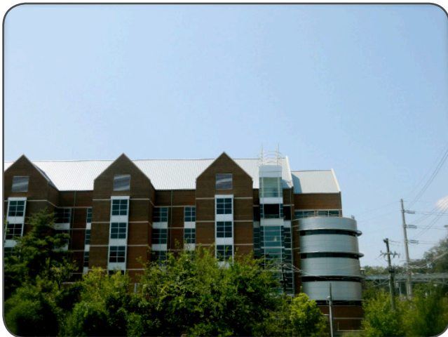
Above: Min H. Kao Building and CURENT Headquarters in Knoxville, TN
